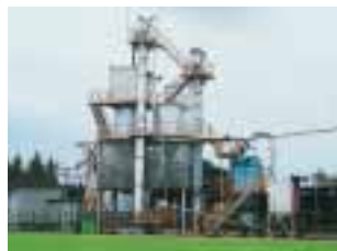
Waste sand recycler at the Moka Works
