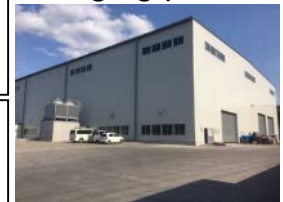
New building for structural steel castings
