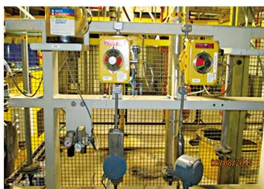
Fig. 4 Chemical flow meters
